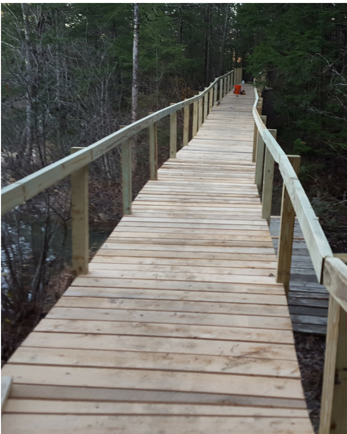
New family friendly bridge at Hawkes Preserve
